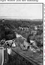
These inclines consisted of 10 and 13 ton cars moving up and down the hill;
